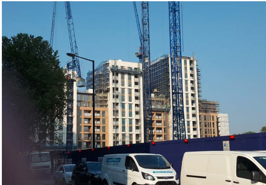
Hermitage Street (front) elevation (top) and rear elevation seen from North Wharf Road (bottom).
